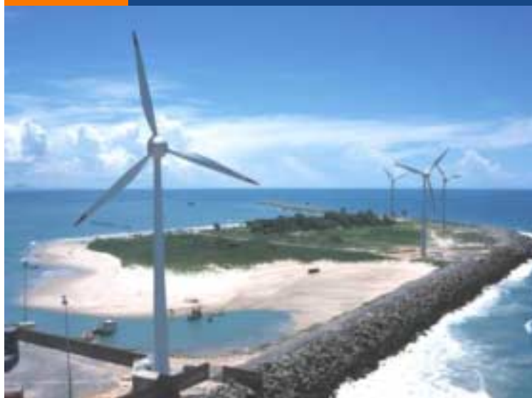
FIGURA 6.12 Central Eólica Mucuripe (Fortaleza – CE)
